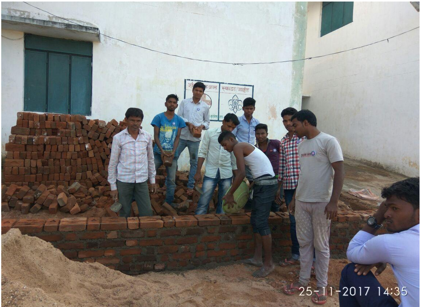
Platform construction in the premises of government higher secondary school Kudakel
