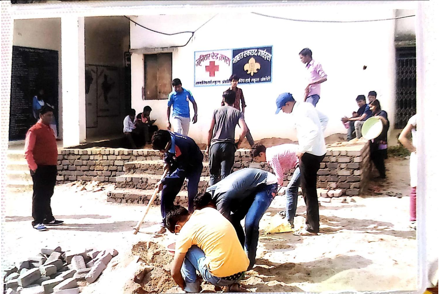
Platform construction at Government High School Premises Aankori
